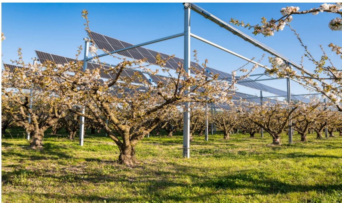
Figure 3 - Interspace Crop-PV installation (SUN'AGRI in SolarPower Europe, 2024b)
