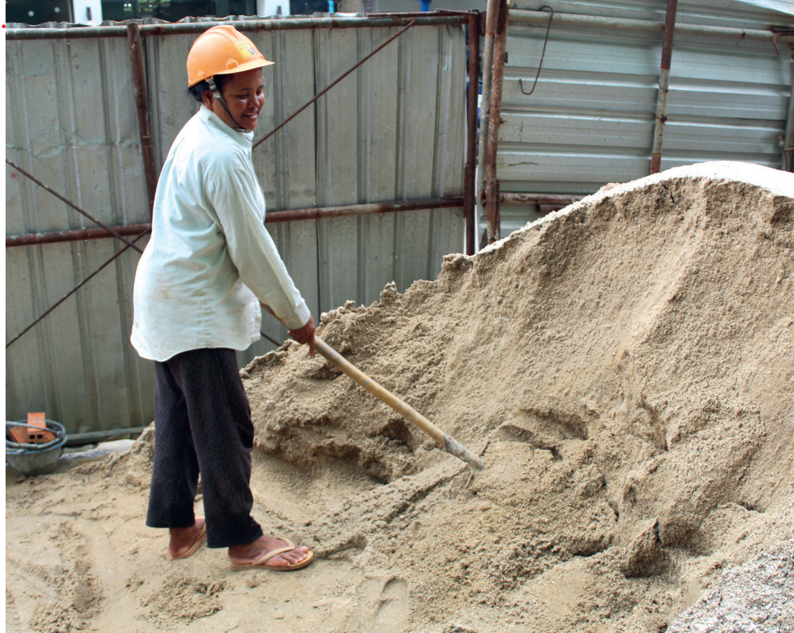
Mrs. Kroeun, working at the construction site.
