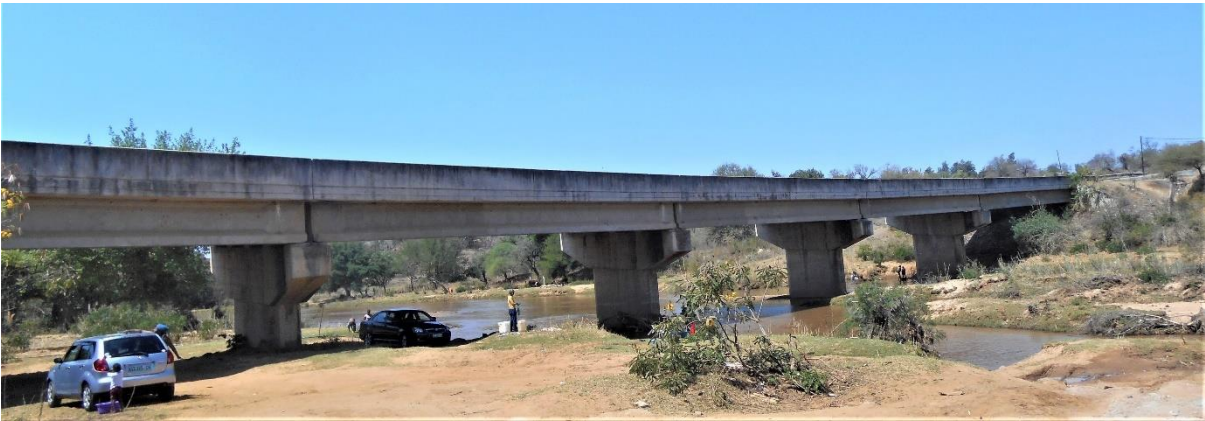
Figure 16 Bridge across the Mbuluzi River financed by the EU.
