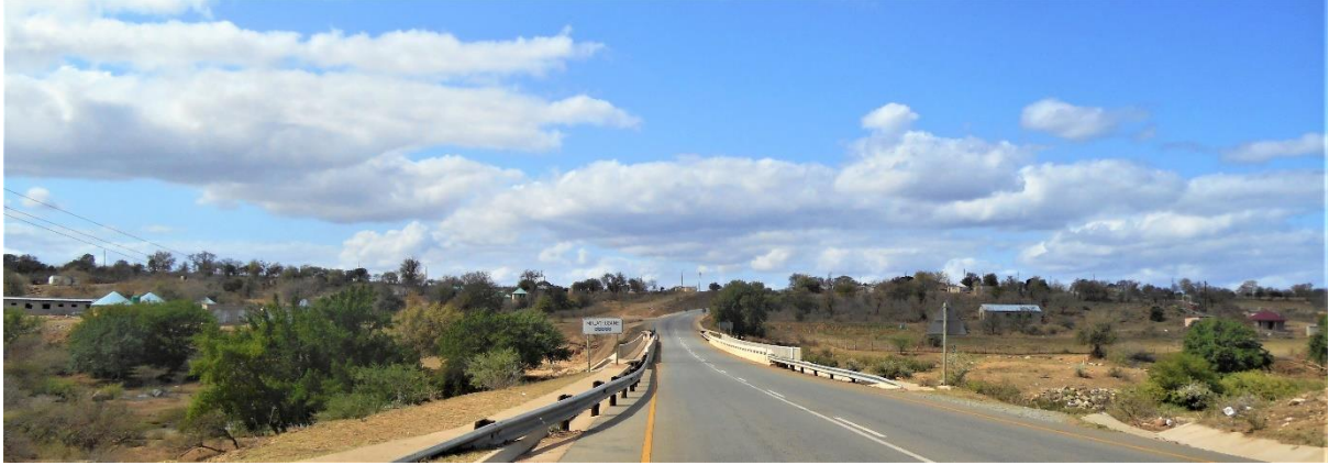
Figure 7 Resurfaced road towards St Philips
