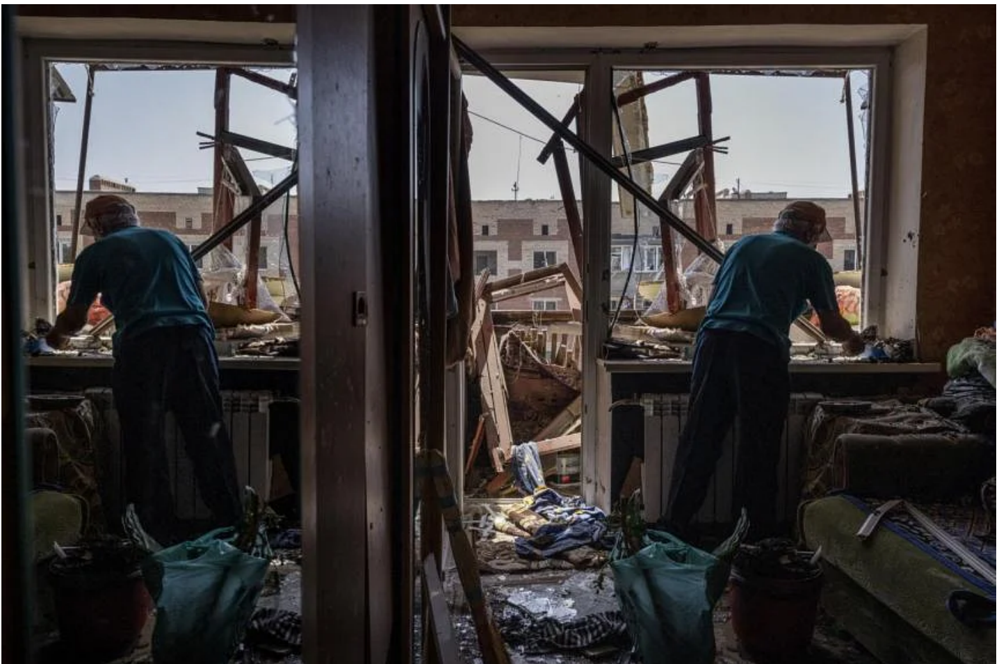
A photo from May 31 showing damage from a Russian missile strike in a residential area in Sloviansk, Ukraine. PHOTO: NYTIMES
