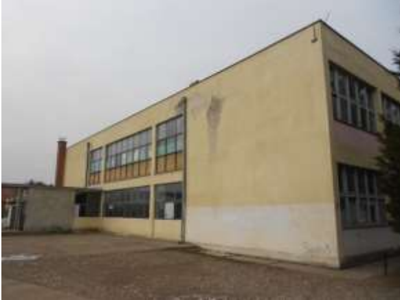
Figure 1: Side & Rear Facade
