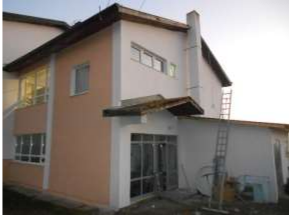
Figure 22: Rear Façade and Boiler room
