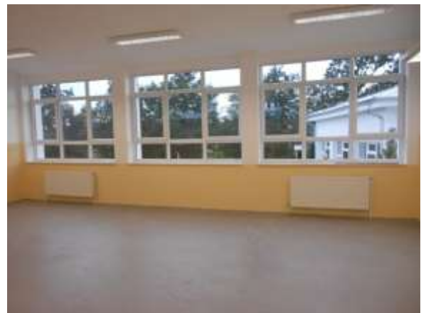
Figure 4: New radiator and refurbished installation
