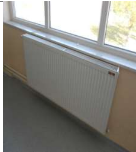
Figure 4: New radiator and refurbished installation
