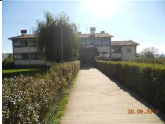
Figure 19: Front and Side Facade Mechanical Installations
