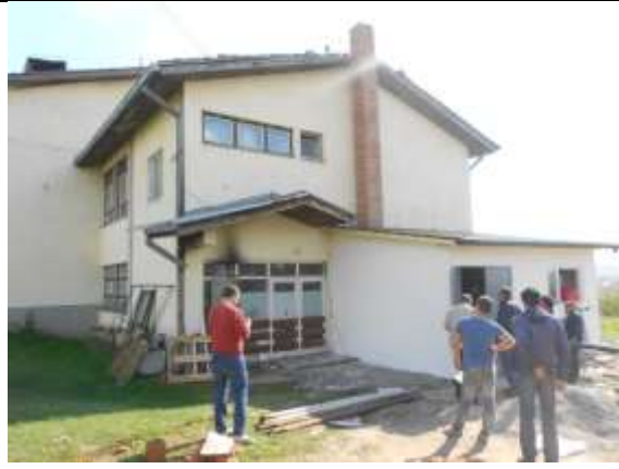
Figure 20: existing Annex and boiler room
