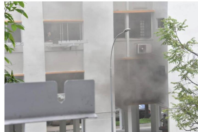
The fire involved a ceiling fan in the living room of a unit in Block 113 Bishan Street 12. PHOTO: ST READER
