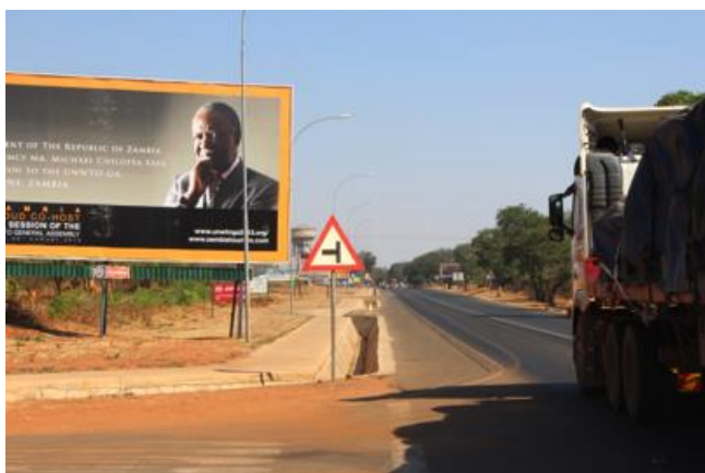
View of project road at road over rail bridge
