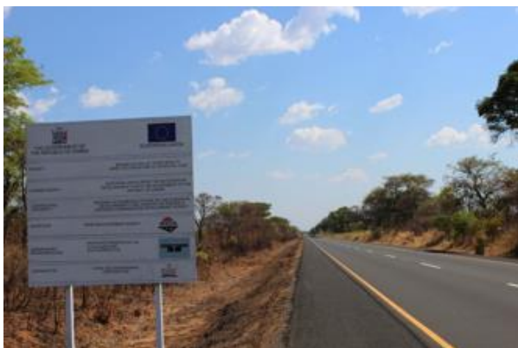
Project signboard at start of 42.8 kilometre section
